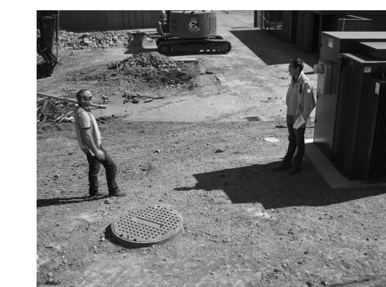
1.1A SWITCHBOARD RELOCATING
