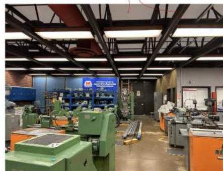
ENHANCED STRATEGY STRUCTURE & CEILING CONDITION
