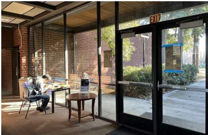
Figure 5.4.1.2.1 - Existing Exterior Storefront
