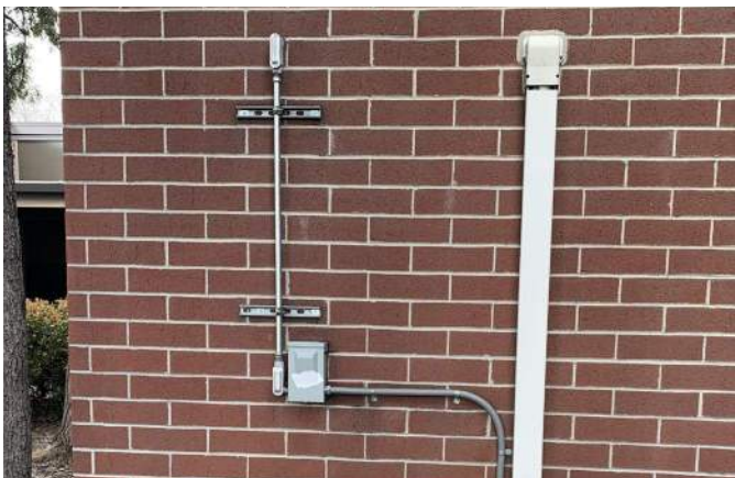
Figure 5.4.1.1.2 - Exterior ET Building's Brick
