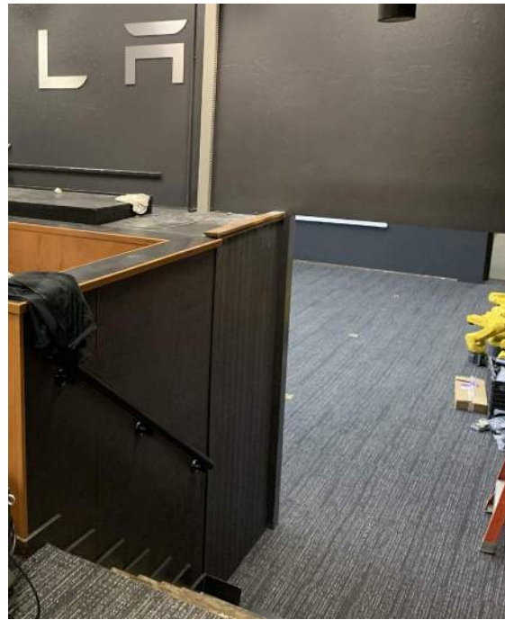
Figure 5.4.2.1.2 - Stairs inside Tesla Lab
