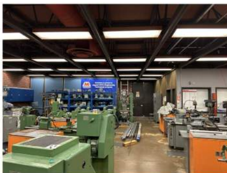
EXISTING EXPOSED STRUCTURE & CEILING CONDITION
