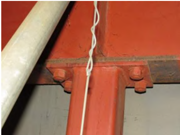
Photo 15: Beam-to-column connection and stiffener.
