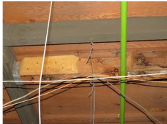
Photo 12: Additional wood blocking.
