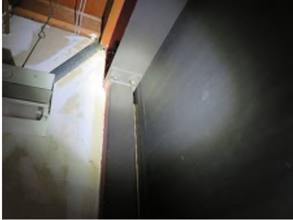
Photo 13: Beam-to-column connection (grid line 15a).
