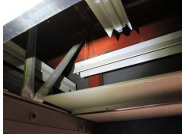
Photo 14: Steel framing along grid line 5.
