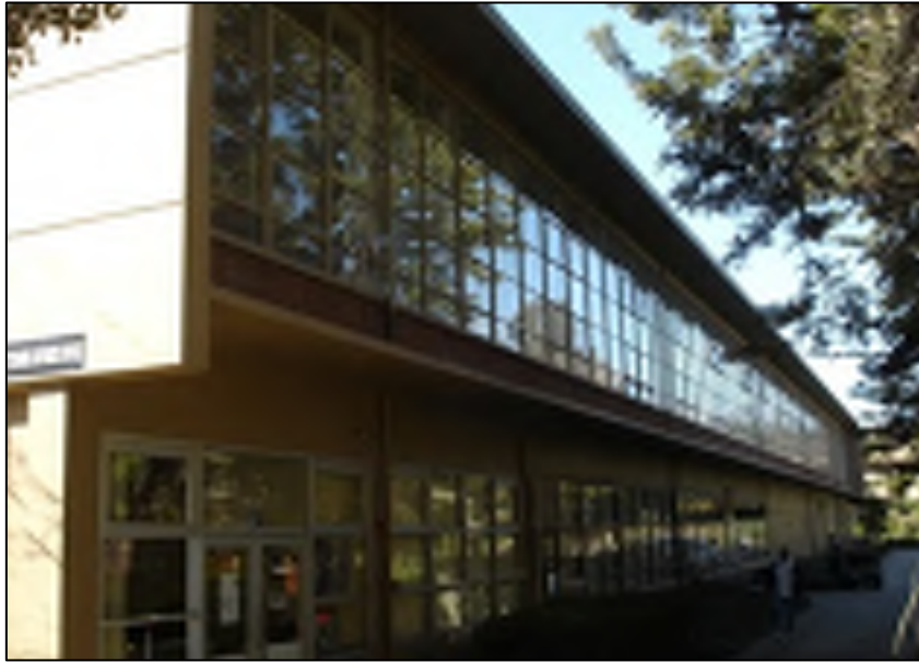
Figure 4: Business Education Building, east faced, view north.
