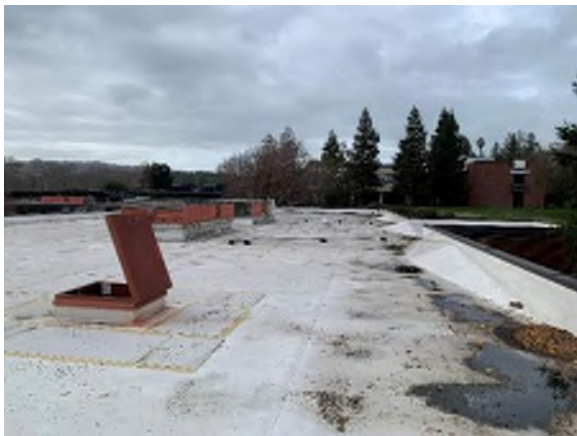
Photo 21: Overall condition of the North Building roof
