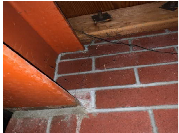
Photo 16: Wide flange beam at transverse shear wall.
