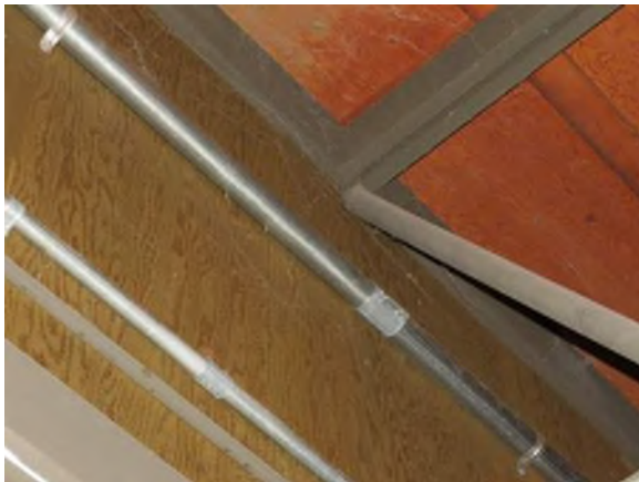
Photo 3: Perimeter wall extending to upper chord of joist.
