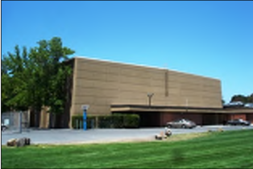
Figure 9: Gymnasium Building, east façade, view west.
