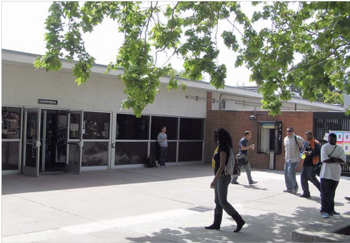
View looking southeast of Cafeteria building
