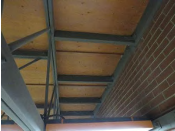
Photo 7: Blocking between joist and parallel shear wall.
