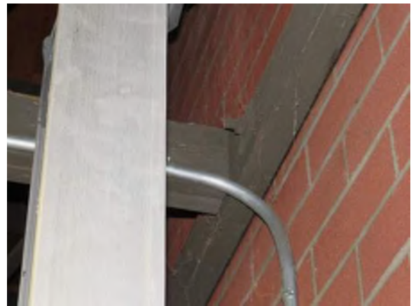
Photo 6: Lower chord joist connection to shear wall.
