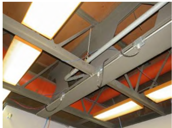
Photo 10: Transfer steel girder.
