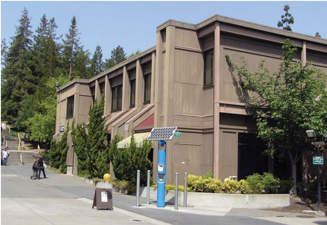
View looking north of the Learning Center
