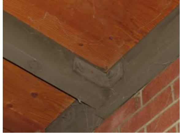
Photo 8: L-clip connecting blocking and shear wall.
