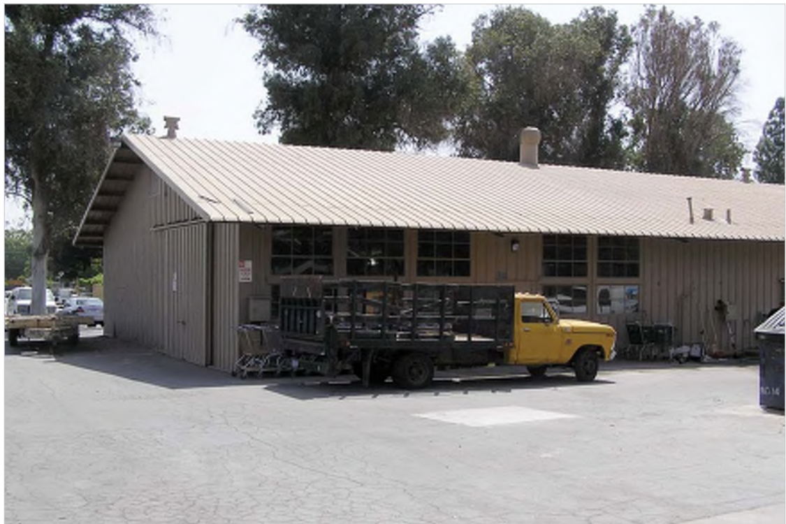
View looking west of the District Storage Building
