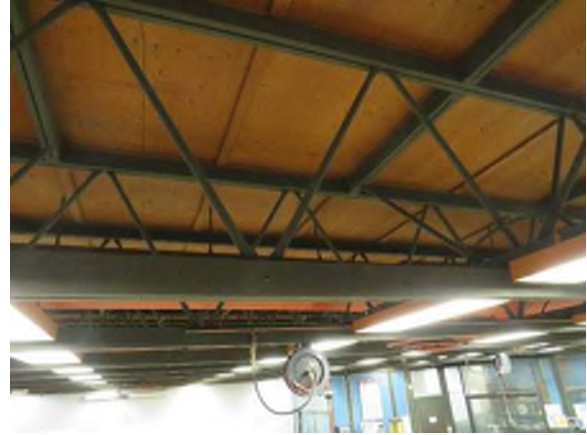
Photo 2: Truss roof joists in north-south direction.
