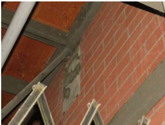
Photo 5: Upper chord joist connection to south shear wall.
