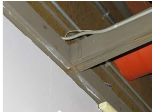
Photo 4: Attachment of lower chord to masonry wall.
