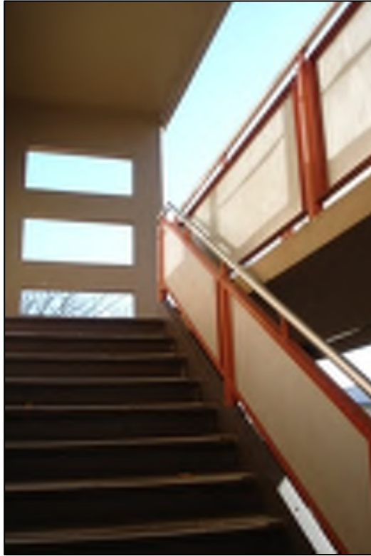
Figure 7: Business Education Building, south stairs, view south.
