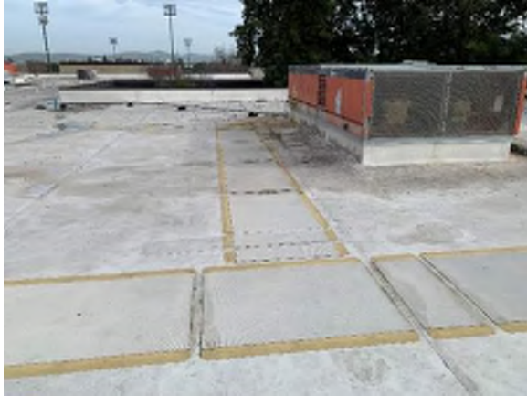
Photo 19: Overall condition of the South Building roof.
