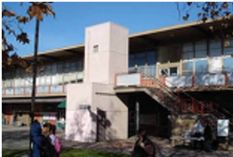
Figure 8: Business Education building, modern elevator addition, west façade, view east.
