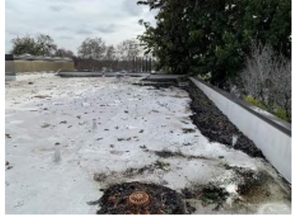
Photo 20: Overall condition of the South Building roof.
