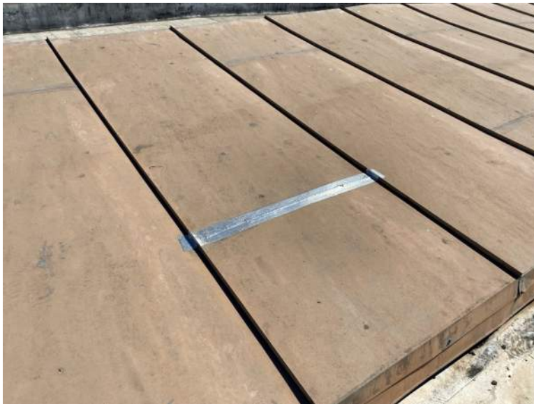
Figure 10. Aluminum-faced tape installed over lap seam joint in metal standing seam roof.
