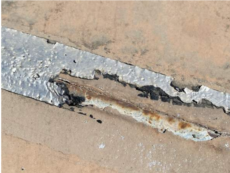
Figure 11. Corrosion observed at the lap seam condition where the aluminum faced tape has deteriorated.
