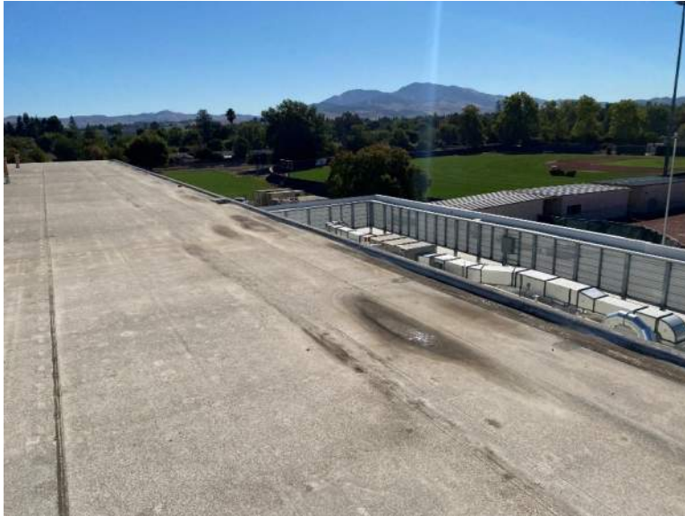
Figure 5. Ponding stains commonly observed within six feet of gutters along PVC membrane seams.
