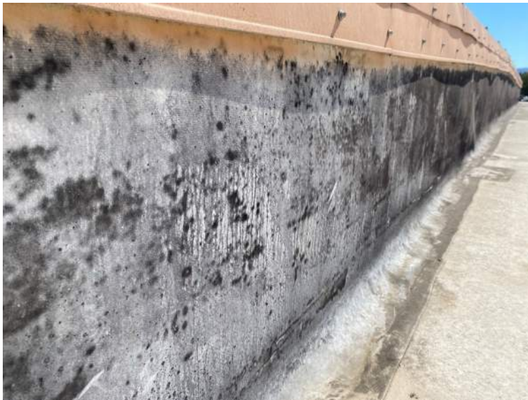
Figure 6. Biological growth is common on the vertical PVC application at the skylight vaults.
