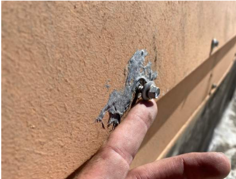
Figure 13. Disengaged fastener at the base of the metal standing seam roof with failed sealant.
