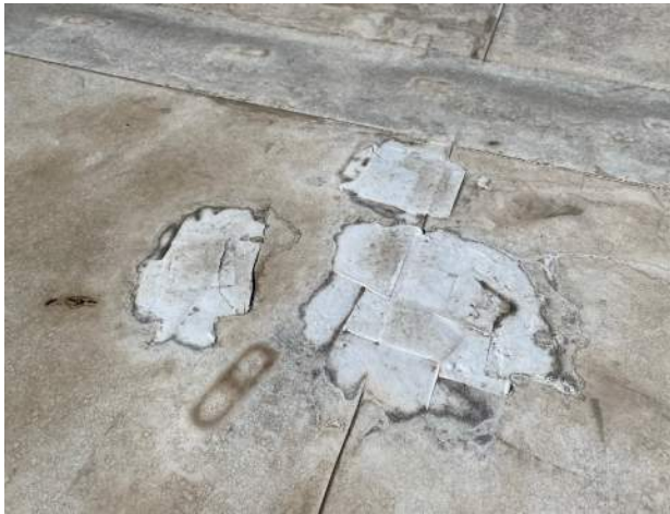
Figure 3. Sealant repair patch over PVC membrane at main roof.
