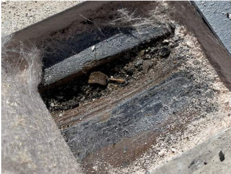
Figure 8. Thin black membrane is installed over the work plank roof deck.
