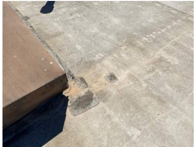
Figure 4. Corner detail patch and repair patch at main roof.
