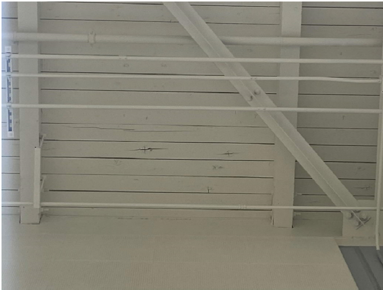
Figure 18. Underside of wood plank roof deck.
