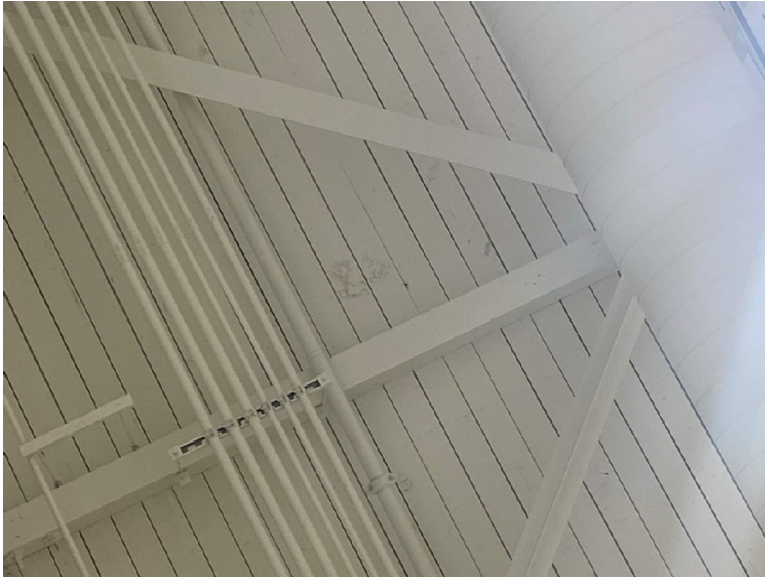
Figure 19. Paint peeling at the underside of the wood plank roof deck.
