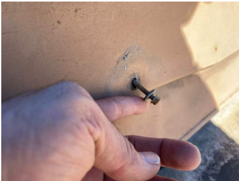
Figure 12. Disengaged fastener at the base of the metal standing seam roof.
