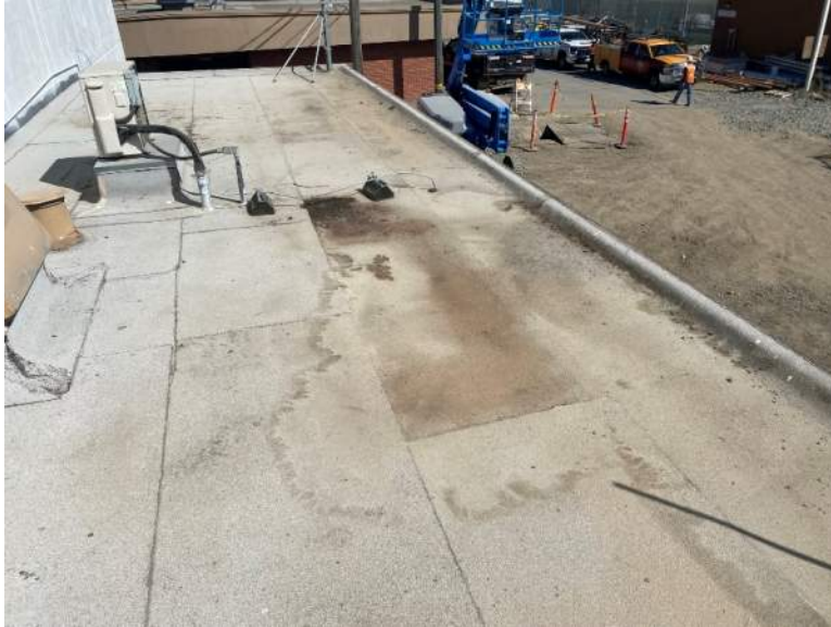
Figure 15. Moisture staining across the outer edge of the built-up roof membrane.
