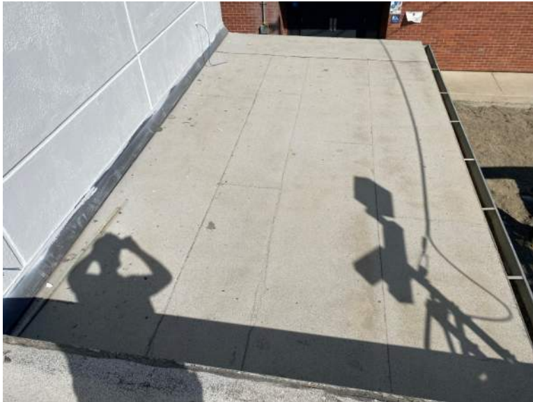
Figure 16. Overall view of lower canopy roof. Roof gutter spans the east edge of the roof.
