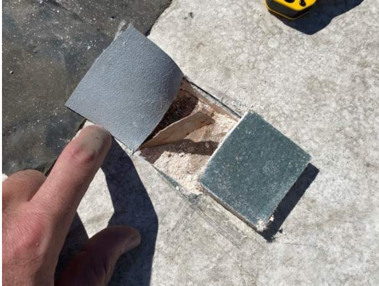
Figure 7. Roof core made at gymnasium main roof.
