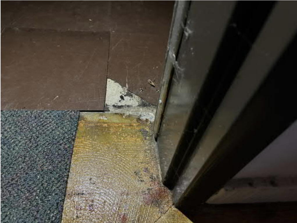
PS Buildings - 12 inch Brown VFT with Black ACM Mastic
