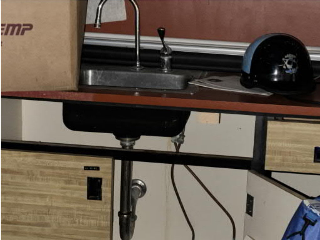
PS Buildings - Black Sink Undercoating
