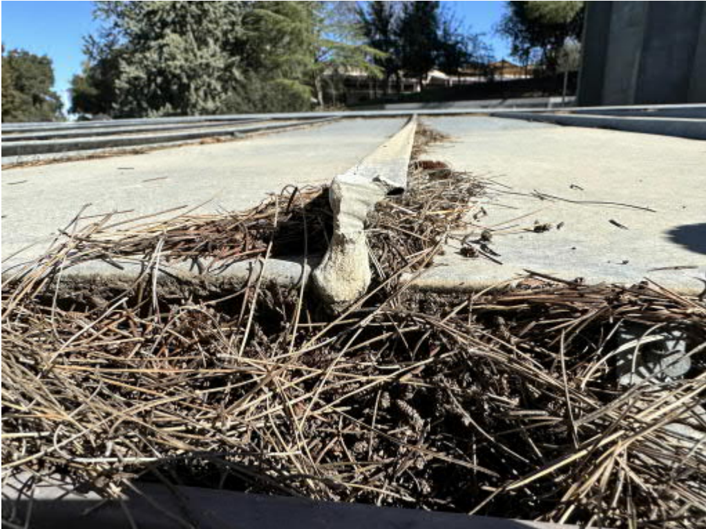
Honors Trailer - Grey Sealant at Metal Roof Edges and Ridge Line
