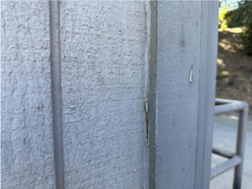
Honors Trailer - Building Caulking at Wood Joints
